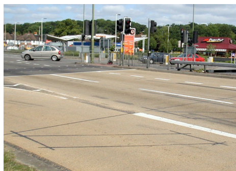
Figura 38 – Bucle inductive instalate in asfalt (exemplu)
