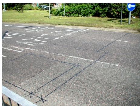
Figura 38 – Bucle inductive instalate in asfalt (exemplu)
